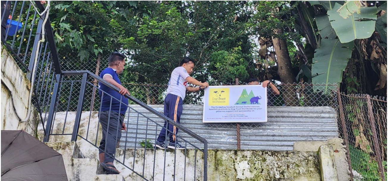
Fig 59: Putting up of sign board after completion of fencing the enrichment zone
